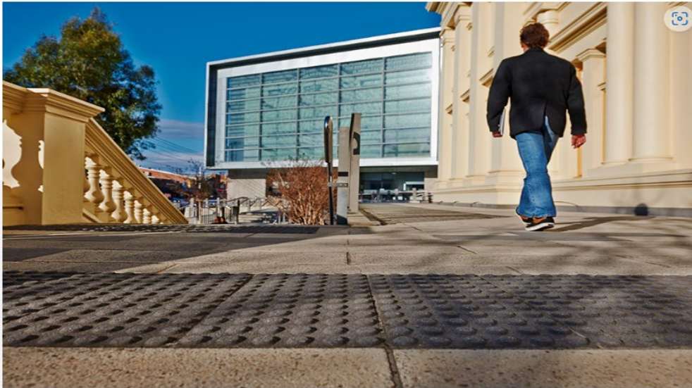
Figure 4.4 Tactile Ground Surface Indicators example (TGSI's)
