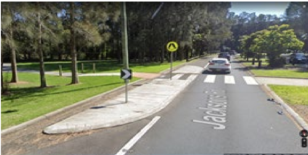
Figure 4.5 Kerb blisters, Jacksons Road, North Narrabeen
