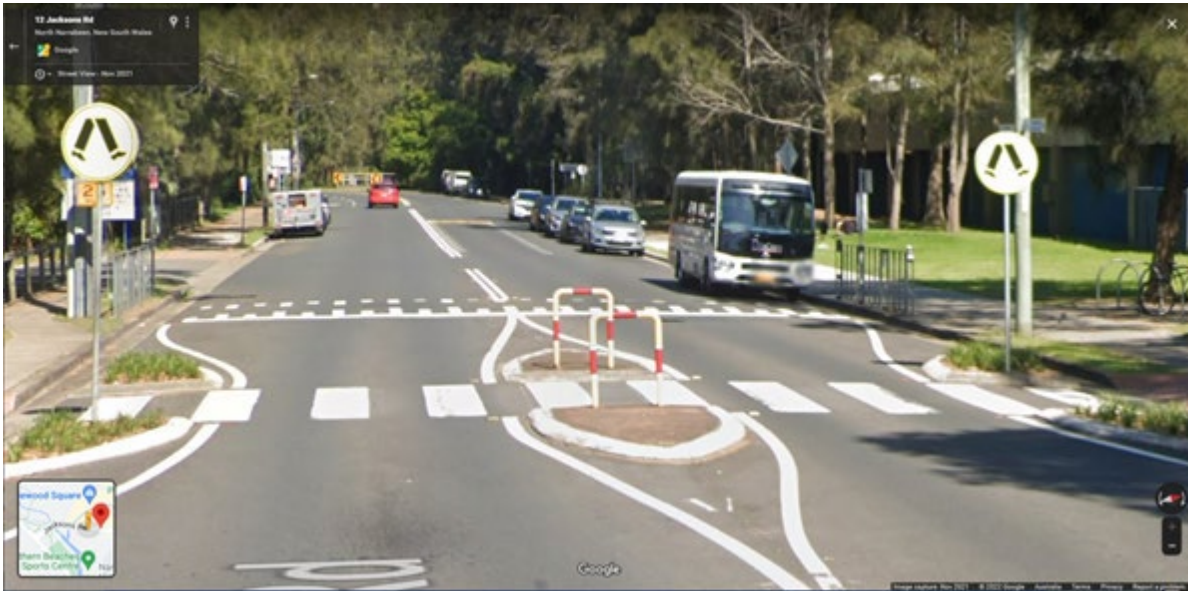
Figure 4.2 Pedestrian crossing with refuge, Jacksons Road, North Narrabeen. Refuges are often supplemented with kerb blisters or extensions
